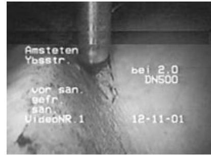
Figure 3 :: An area of inward folding being cut out remotely.
