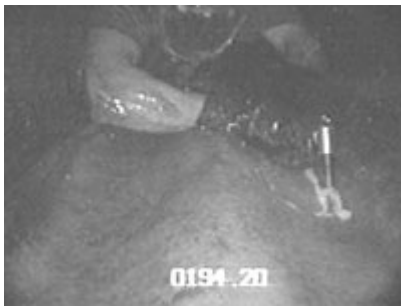
Figure 4 :: An area of inward folding being cut out by hand.
