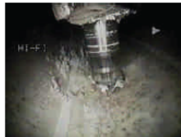
Figure 2 :: Spots associated with a change of section (e.g. manhole).
