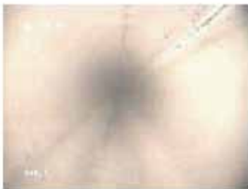
Figure 1 :: Small dark stains on seams.
