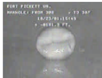
Figure 2 :: Example of stuck inversion with a split plain inner, or flame bonded across the inner layer.
